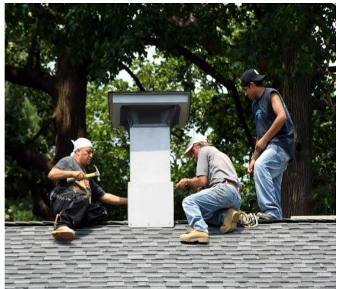
Workers from George Haag Construction Co. install a chimney vent on the roof peak of Maywood Station on July 3, 2006. The chimney vent was fabricated to replicate one that was originally found on Maywood Station in the 1872 to 1920's period. (Photo by Ed Kaminski)
