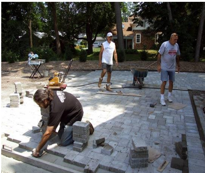
On July 3, 2006 masons from A. Lepore & Grandson Masonry completed Phase 2 of the installation of Brussels Blocks on the station grounds. The blocks now cover the driveway side of the station and connect to Maywood Station's Caboose 24542 further increasing handicap accessibility. (Photo by Ed Kaminski)
