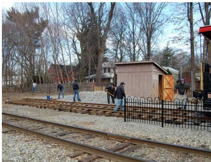
A work session was held on January 27, 2008 to install ballast for the new panel track extension and beautify the grounds including tree trimming, brush cutting and landscaping. (Photo by Keith Smollin)
