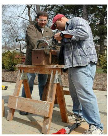
MSHC members Rob Pisani and Hector Hernandez, Jr. work on cutting a profile into the base of one of the two new finials being applied to Maywood Station's end roof peaks at the March 31, 2007 work session. The angle of the profile was very important to ensure and exact fit on the roof peak. (Photo by Doug Earls)
