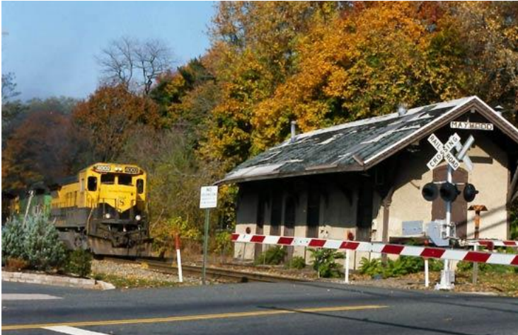
Maywood Station as it appeared in October 2001 as a New York, Susquehanna & Western Railway freight train was approaching. The station was near a state of disrepair and in the process of being reclaimed by nature. (Photo by Keith Smollin)
